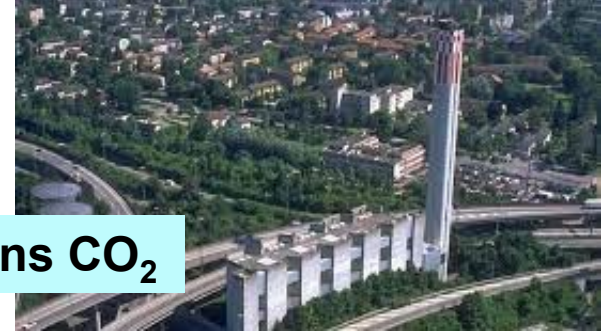
wood-fired energy plant
