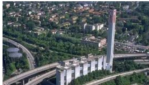
wood-fired energy plant
